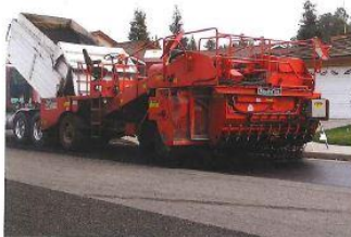
In Clovis, Calif, hot chips are spread on rubberized asphalt in advance of slurry surfacing to complete cape seal
